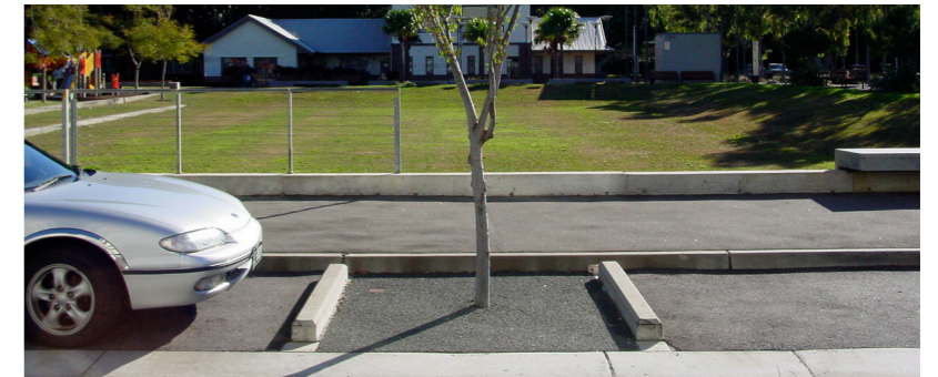
IN VERGE TREE PLANTING BAYS
